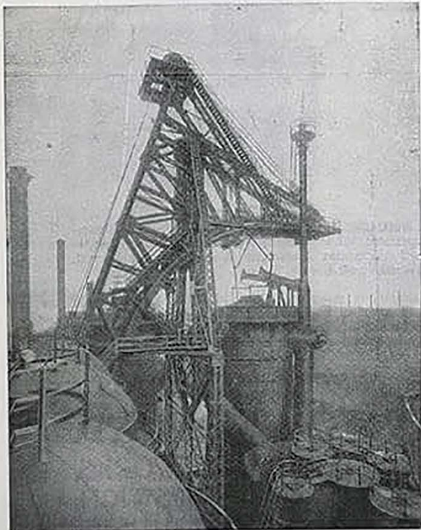
Blast Furnace Charger.
